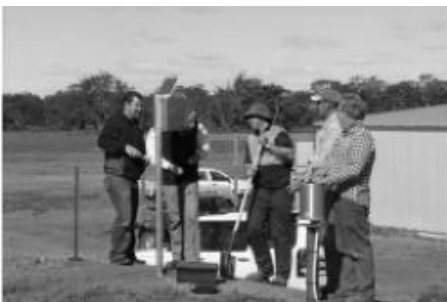
Metering transmitter & telemetry at Old Coree
