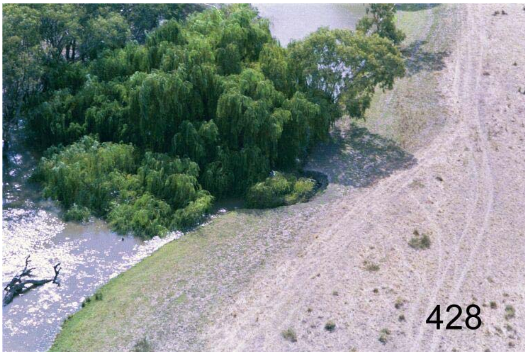
Plate 15: Streambank Erosion caused by willows diverting flow
